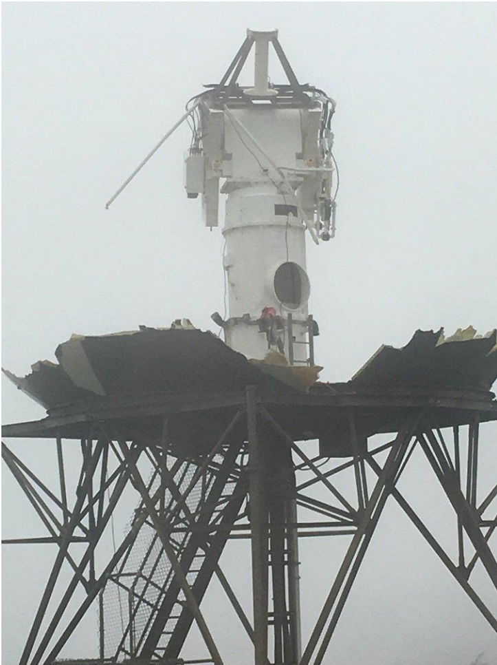
Puerto Rico weather radar destroyed by Hurricane Maria
